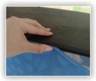
6. Angle and tuck gasket into channel in edge of counter top. Insert graphic gasket all the way around.
